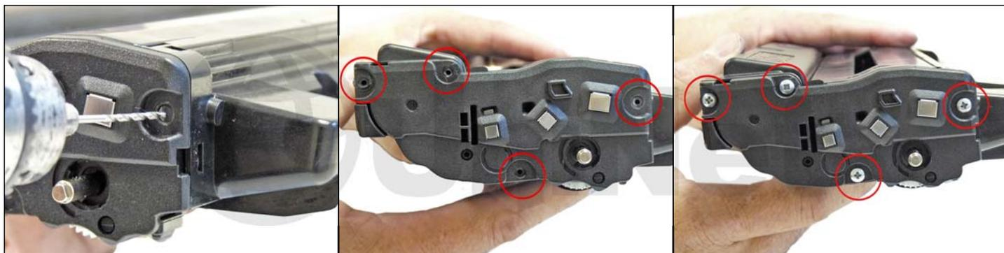
33. Drill four small holes that correspond to the screw size you are using.
